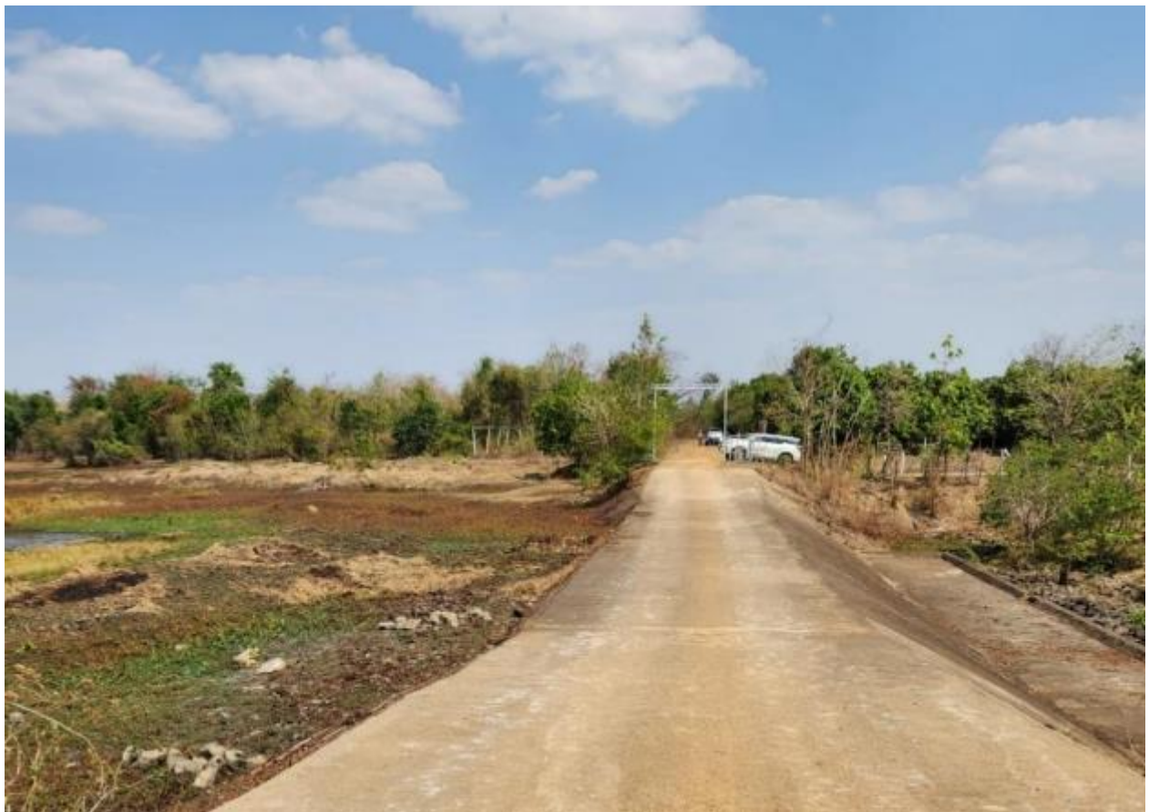
Figure 1 – Overview of Kantout Reservoir (near spillway)
