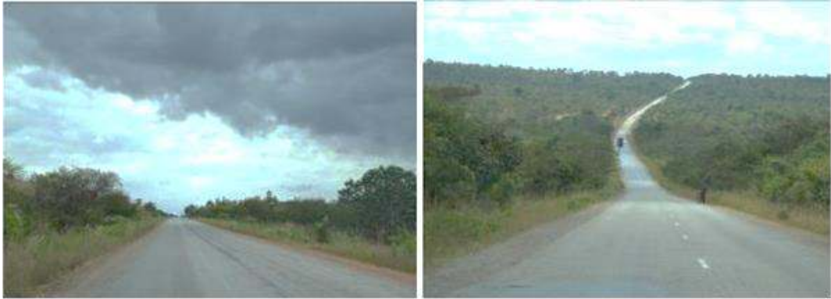
Figure 4-1 Flat (L) and Undulating (R) terrain of the project road
