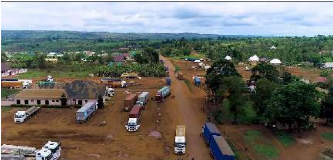
Figure 4-20 Typical truck stop along the road
