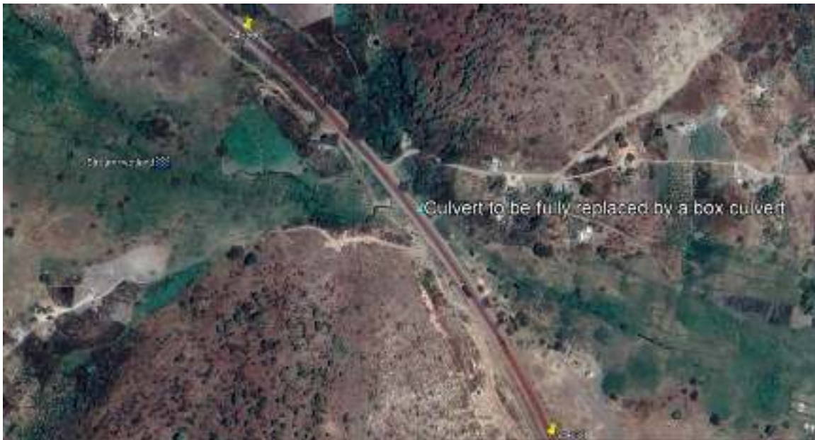
Figure 7-2 Example of a highly sensitive area where pumps and temporary enclosure shall be used to ensure free flow of water
