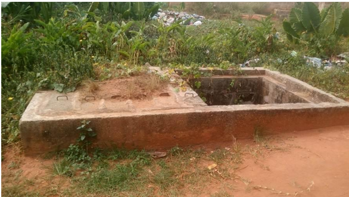
Plate 4.4: Manhole constructed by previous intervention
