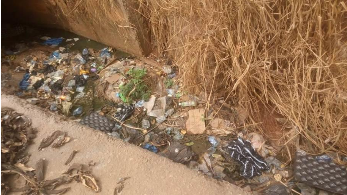
Plate 4.3: Wastes in drainages constructed by previous intervention
