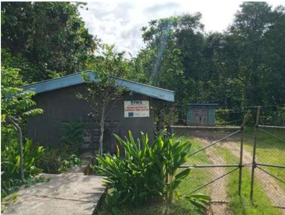
Plate 2: Existing Kongulai Pump Station
