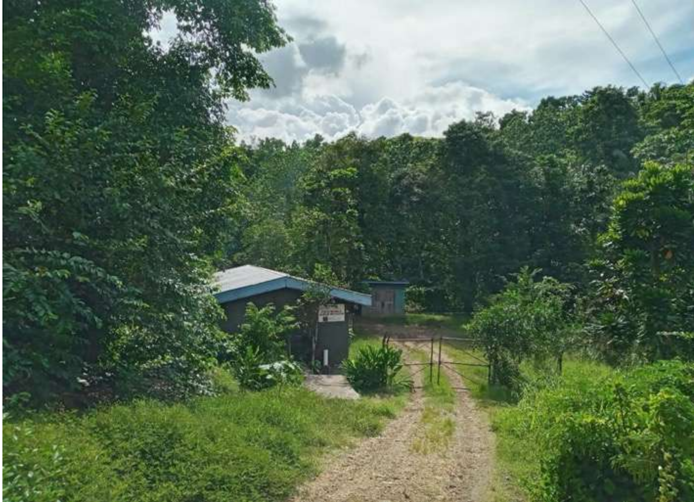
Figure 3: The current Solomon Water Pump Station Site at Kongulai Spring
