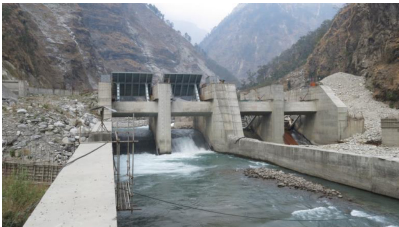
Photo D1.2: Dam Site of UT-3A, 2015
