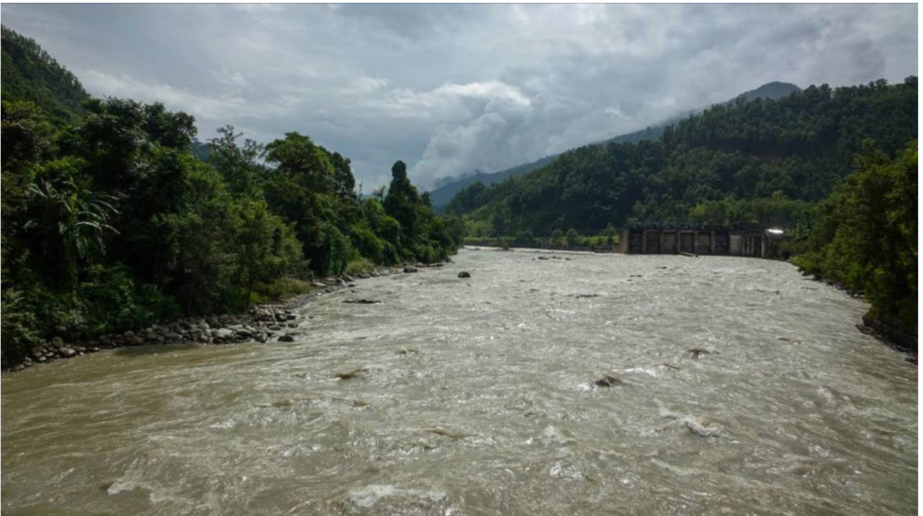
Photo D1.4: View of Existing Trishuli HPP from Upstream, 2016
