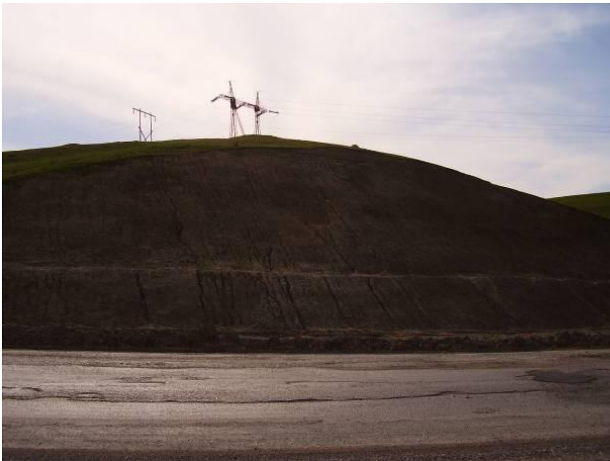
Figure 4-2: Example of Landslide Prone Area along the Study Route
