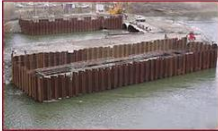
Figure 5.1: Steel sheet pile coffer dam for in-river construction activities
