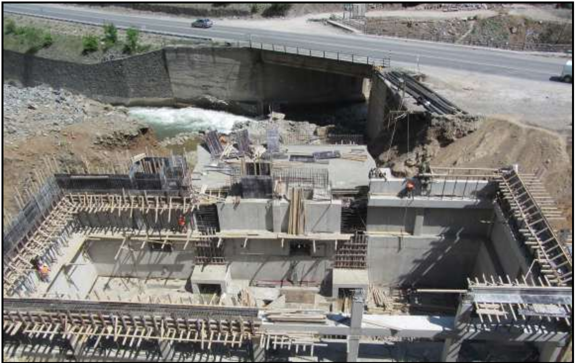
Figure II.4.5. A View from Power House Construction
