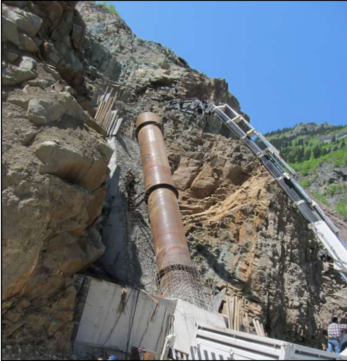
Figure II.4.6. A View from Penstock Pipe Route
