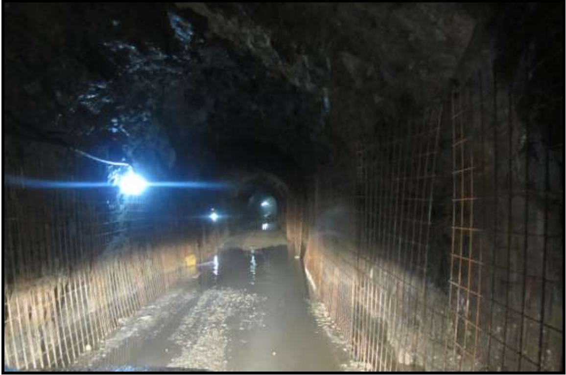
Figure II.4.4. A View from Transmission Tunnel
