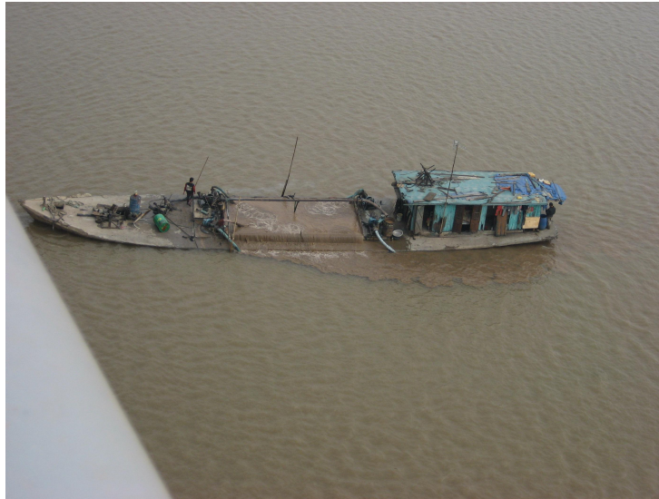
Photo 5-1. Dredging in Red River
