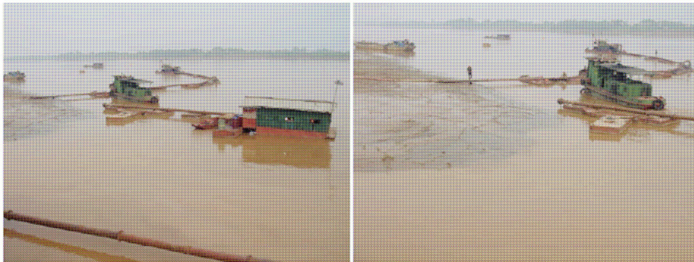
Figure 0-3. Dredging works at Khuyen Luong Port
