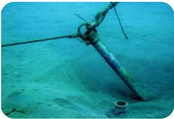
A 2-m long, heavy 5–7 cm diameter galvanized metal pipe hammered diagonally into the seabed being used as an anchor for a floating nursery above a sandy bottom (S. Shafir).
