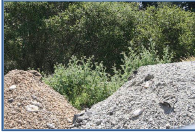
Figure 12. Cover soil stockpiles to prevent invasive plant establishment. Monitor worksites for invasive plants and/or other AIS following activities.
