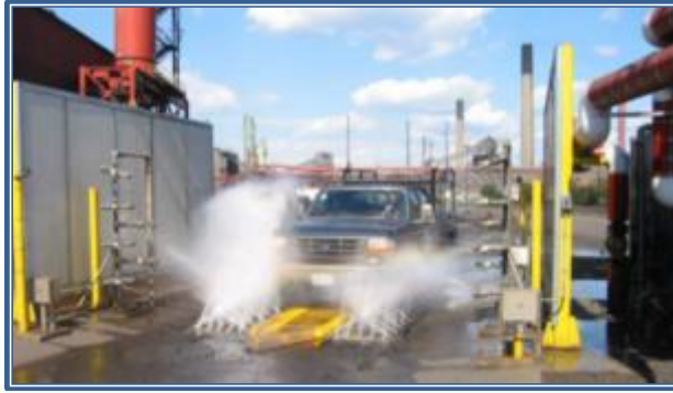
Figure 5. Identifying a facility to properly wash vehicles and equipment is an important step in the prevention of invasive species 9
