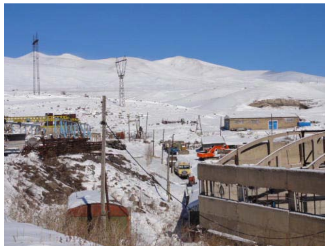
Figure 12-51: Affected building in village Shaki
