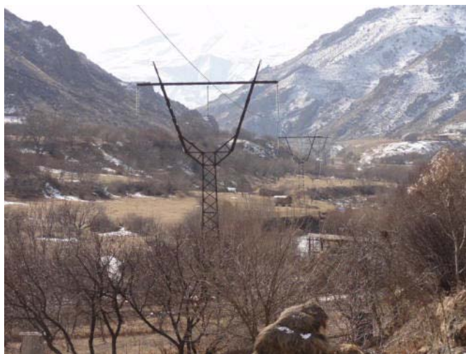
Figure 12-32: Present line below Shatin towards village Getap
