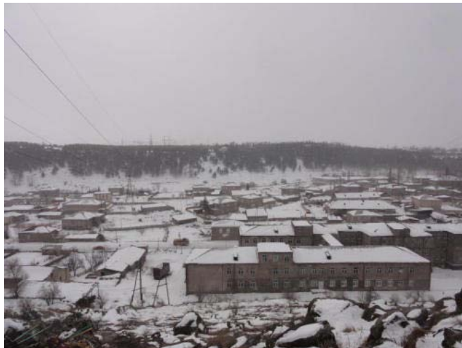
Figure 12-17: Overspanning Valley Gavar
