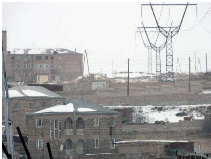
Figure 12-12: Last 3 Towers Noratuz Line before Gavar Substation
