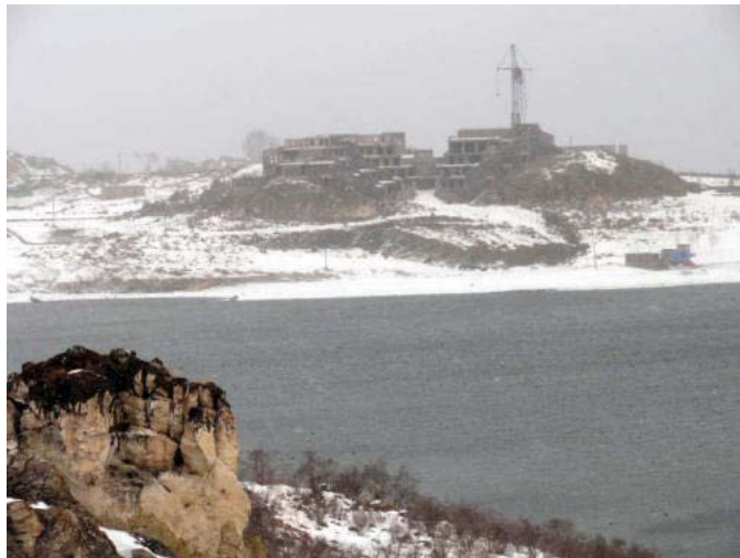
Figure 12-20: Construction on Sevan Lake shore
