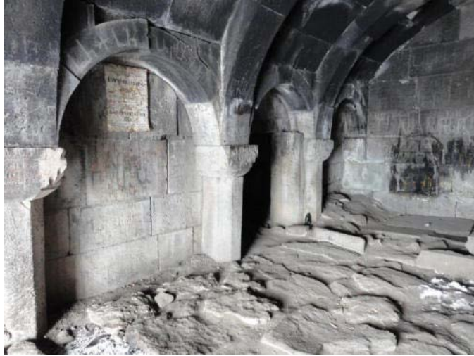
Figure 12-25: Caravanserai on Selim Pass
