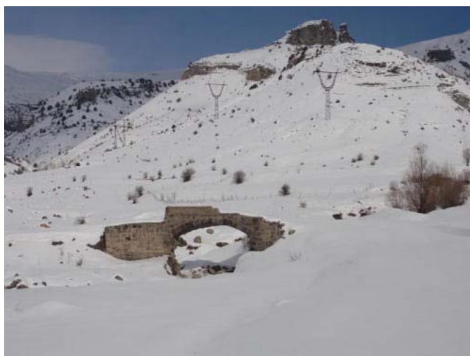
Figure 12-27: Historical Bridges in Yeghegis Valley
