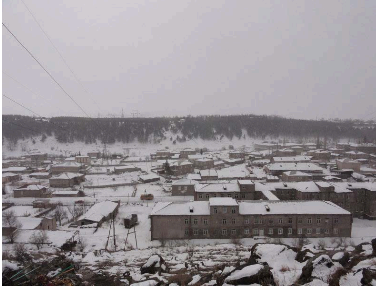
Figure 7-18: Overspanning of Gavar Valley
