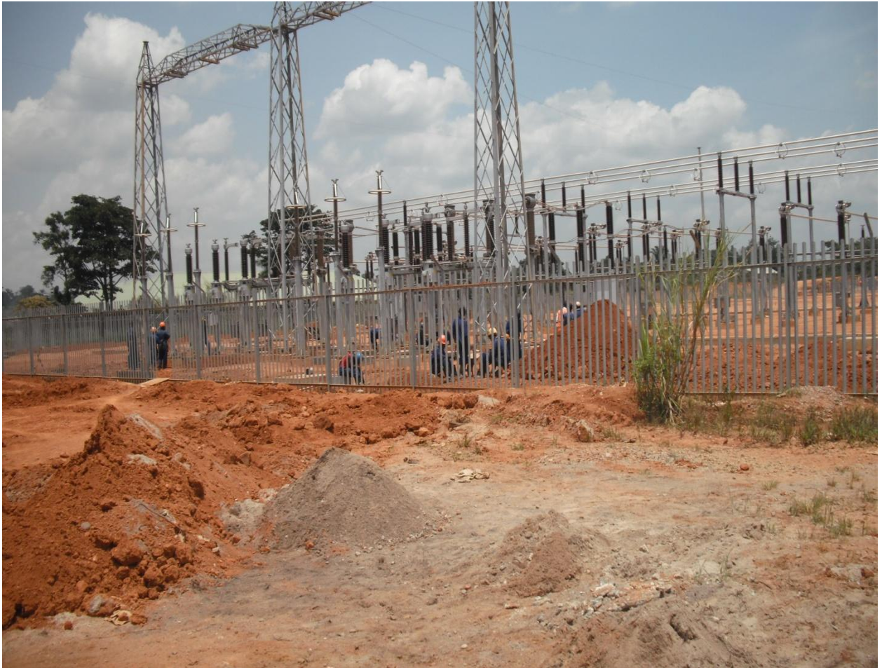
Figure 5: Kawanda Sub Station Under construction
