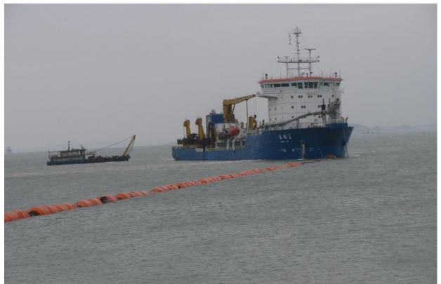
Figure 3.2-4 Hydraulic filling through floating pipe
