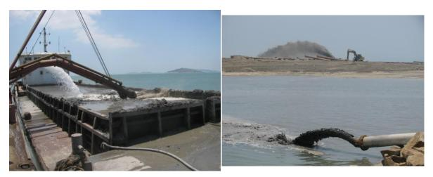
Transfer blowing from the hopper barge
