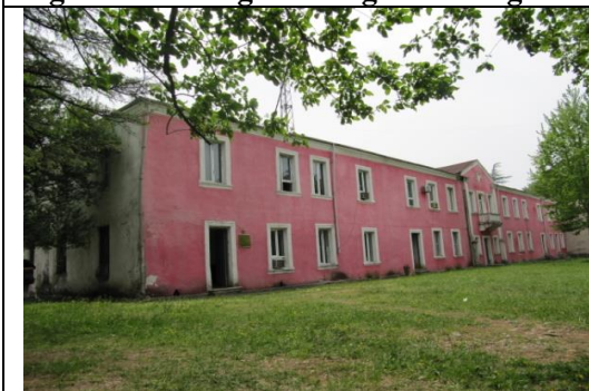
Fig. 3.4. Existing Building of Sakrebulo
