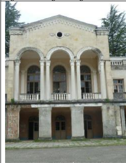
Fig. 3.6. Existing Building of Railway Station
