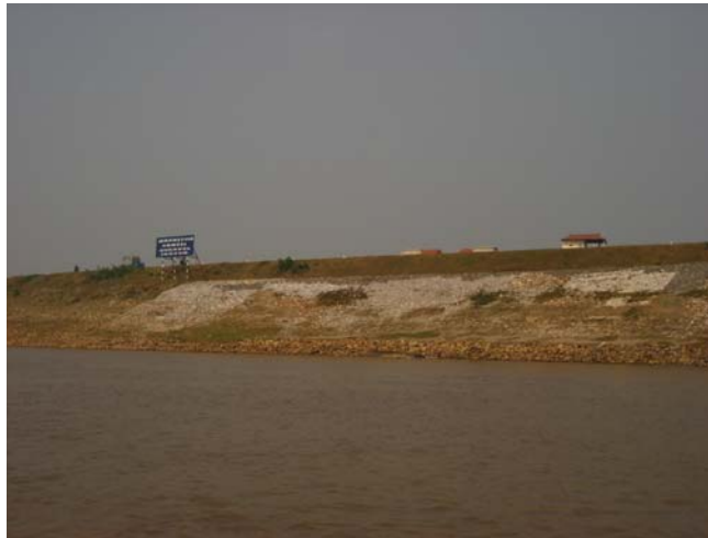
Photo 5-2 Bank Protection in Duong River at About Km 0.
