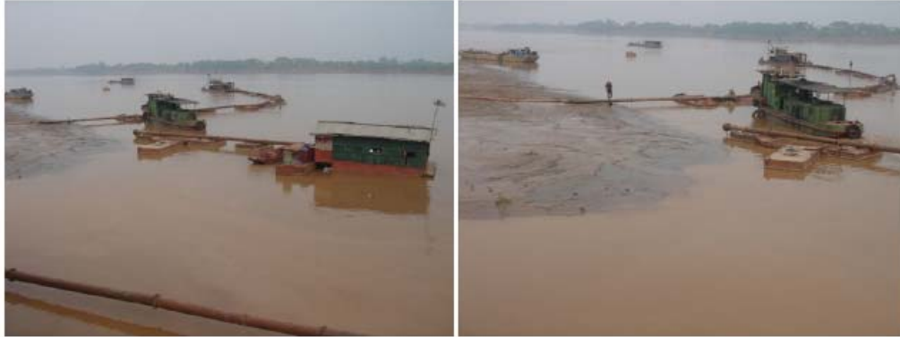
Figure 3-3. Dredging works at Khuyen Luong Port
