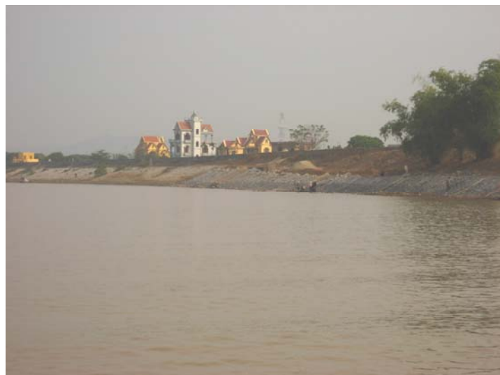
Photo 5-5. Bank Protection Construction in a Segment of Corridor 1.
