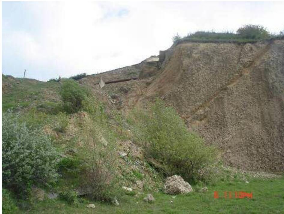
Igoeti. Landslide induced by road construction: site 1
