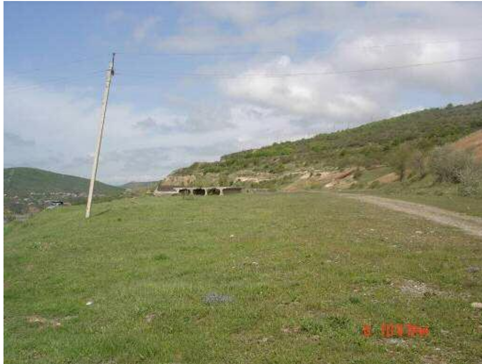
Igoeti. Landslide induced by road construction: site 1
