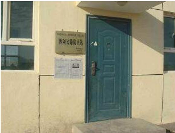
Boa Road Fire Station
