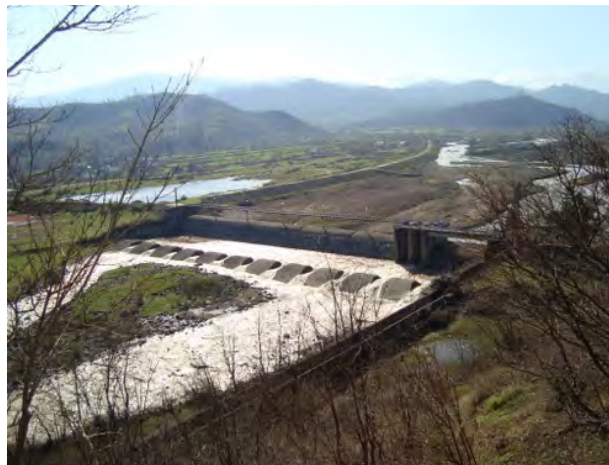
Luveser Dyke on the Lankaranchay river nearby Luveser Village
