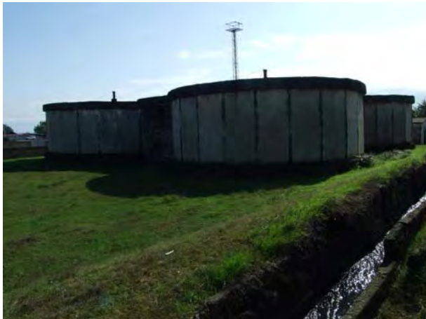
Existing WWTP site
