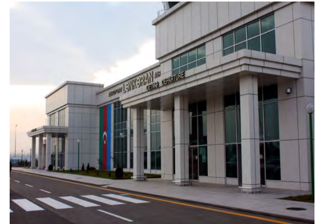
Air Terminal Building
