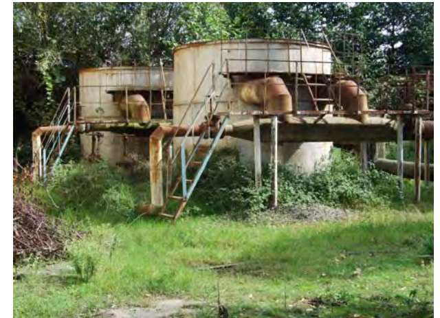
Existing WWTP site North of Goyshaban district
