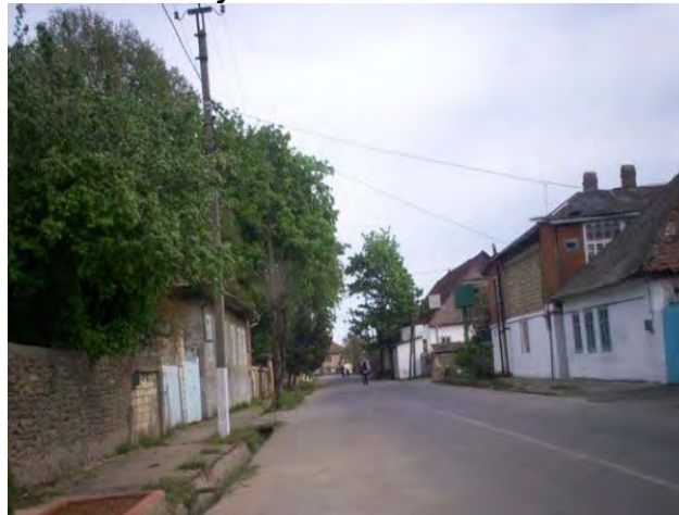
A Street and road side open channel
