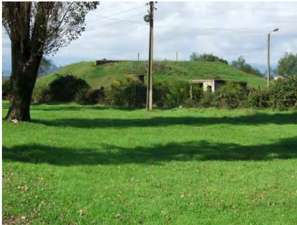
Existing Distribution Reservoir nearby SEF Village
