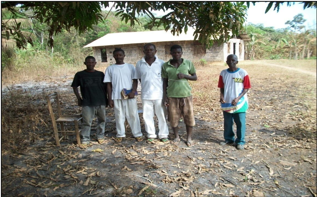
Figure 14 In the back ground sun dried bricks house under construction using Mud (earth) as cement with corrugated sheet roof
