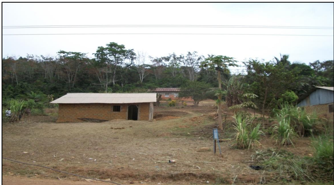
Figure 13 Sun dried bricks house under construction
