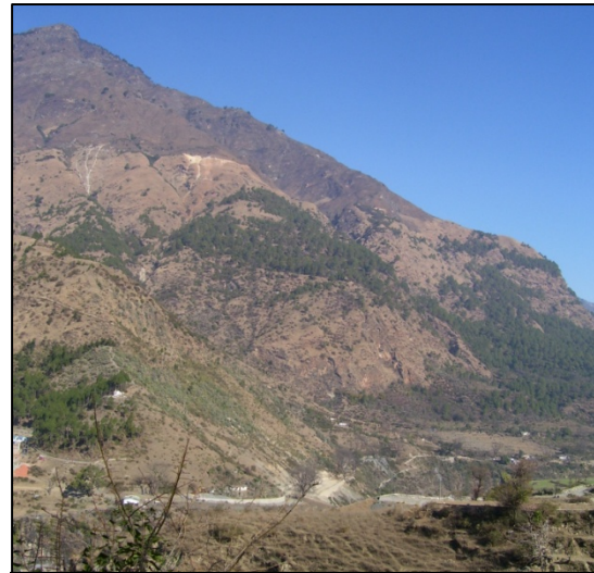
View of Powerhouse site
