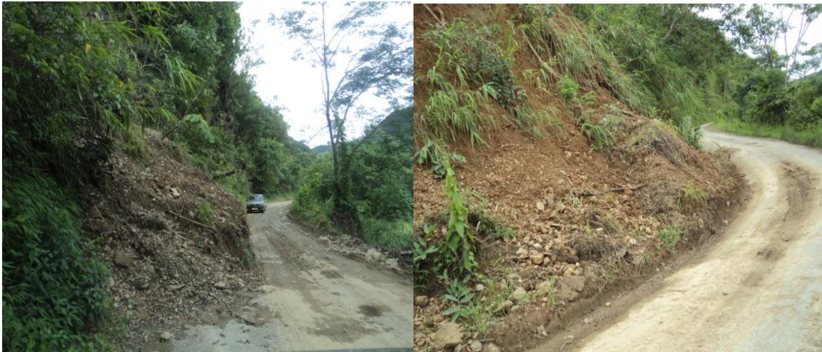
Photographs 2.1 : Landslides along the Champhai Zokhawthar road
