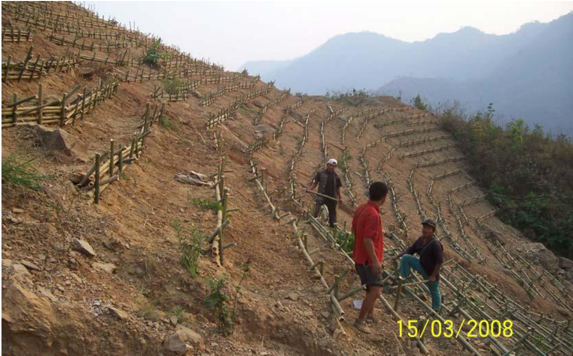
Bamboo crib wall during implementation
