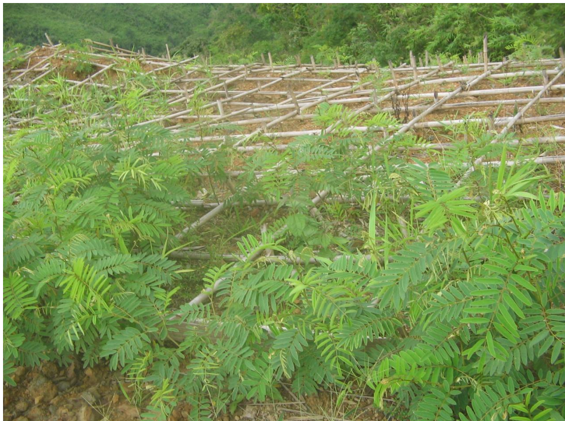
Bamboo mating for potection of disposal site
