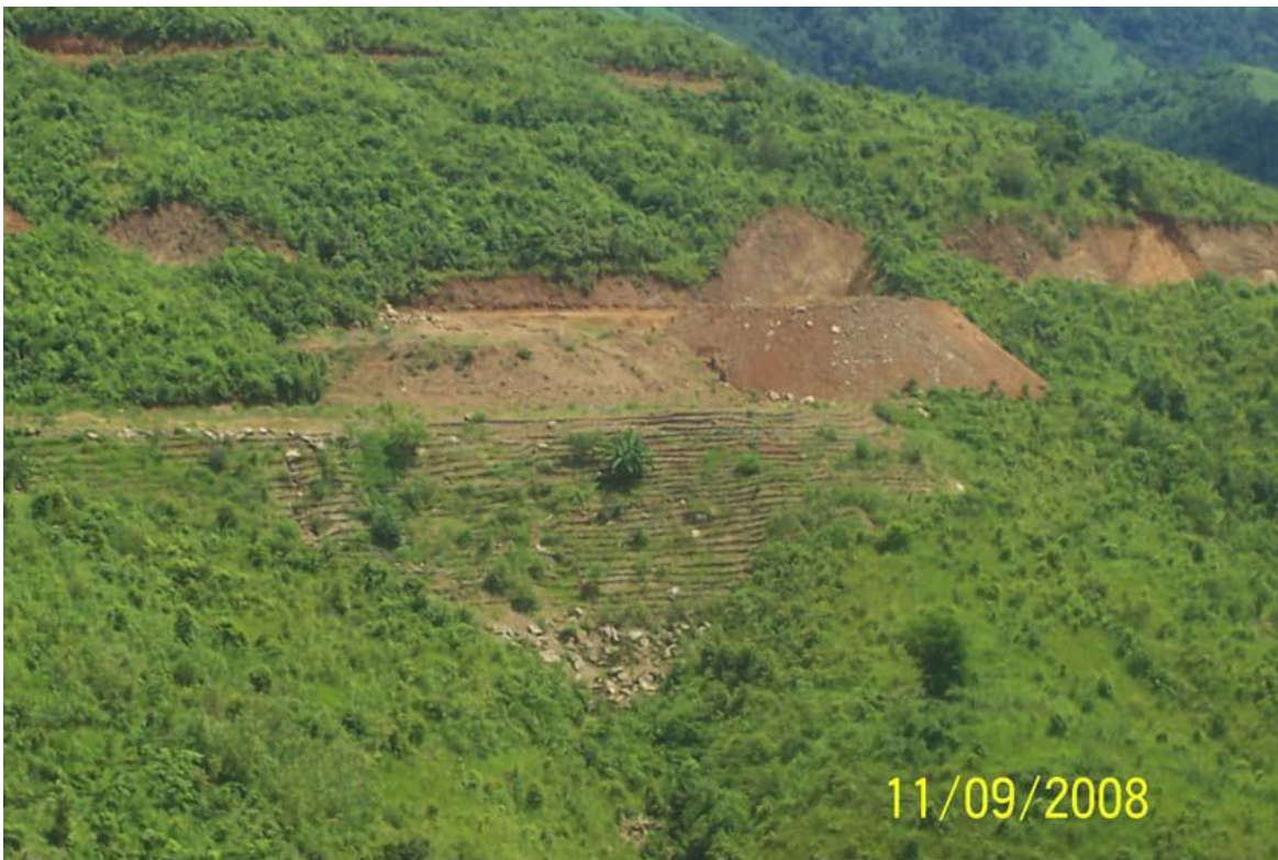
Bamboo crib wall after implementation
