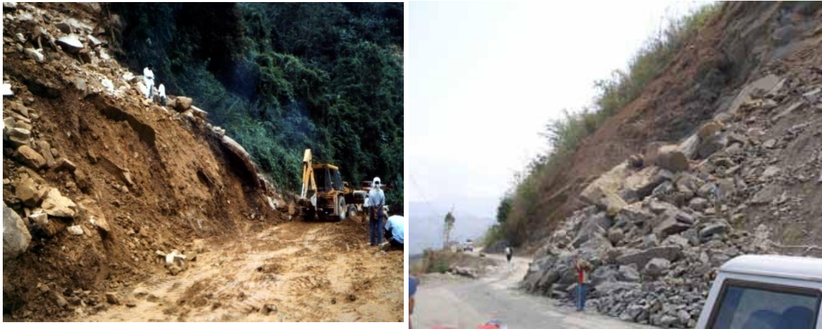
Photographs 3.3: Land slide during construction in some roads in the project region
