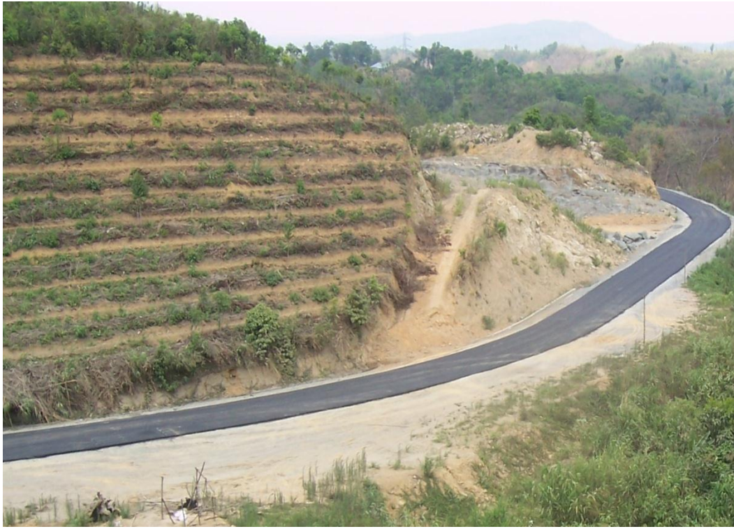
Bamboo matting for potection of slopes
