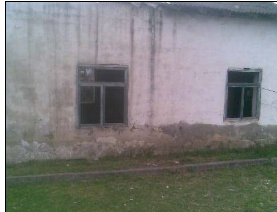
A pump station in Astara city
