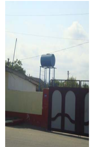
An elevated water reservoir in Astara
