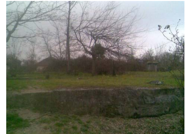
Existing Water reservoir nearby Alasha village
