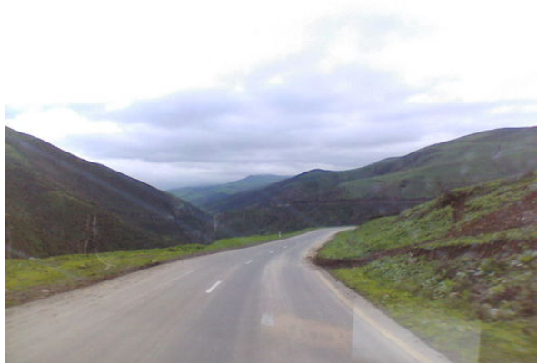
Astara city – Sim village asphalt paved secondary road
