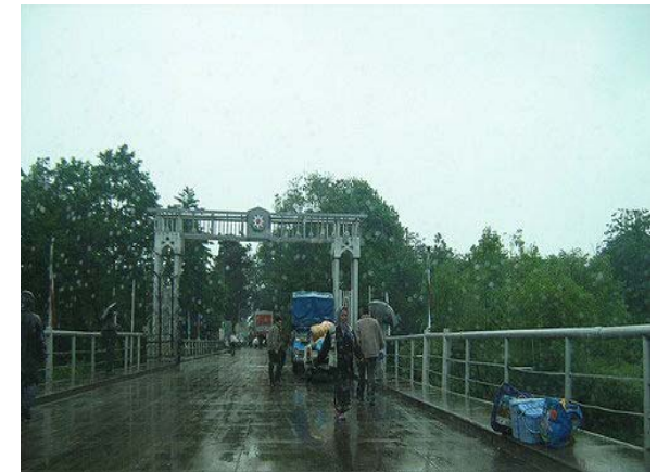
Bridge on Astarchay river, which provides the connection between Azerbaijan and Iran, South of Astara city
