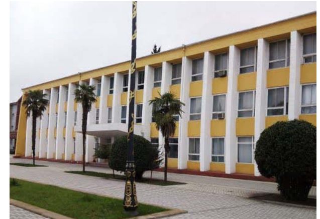
An institutional Building in the city
