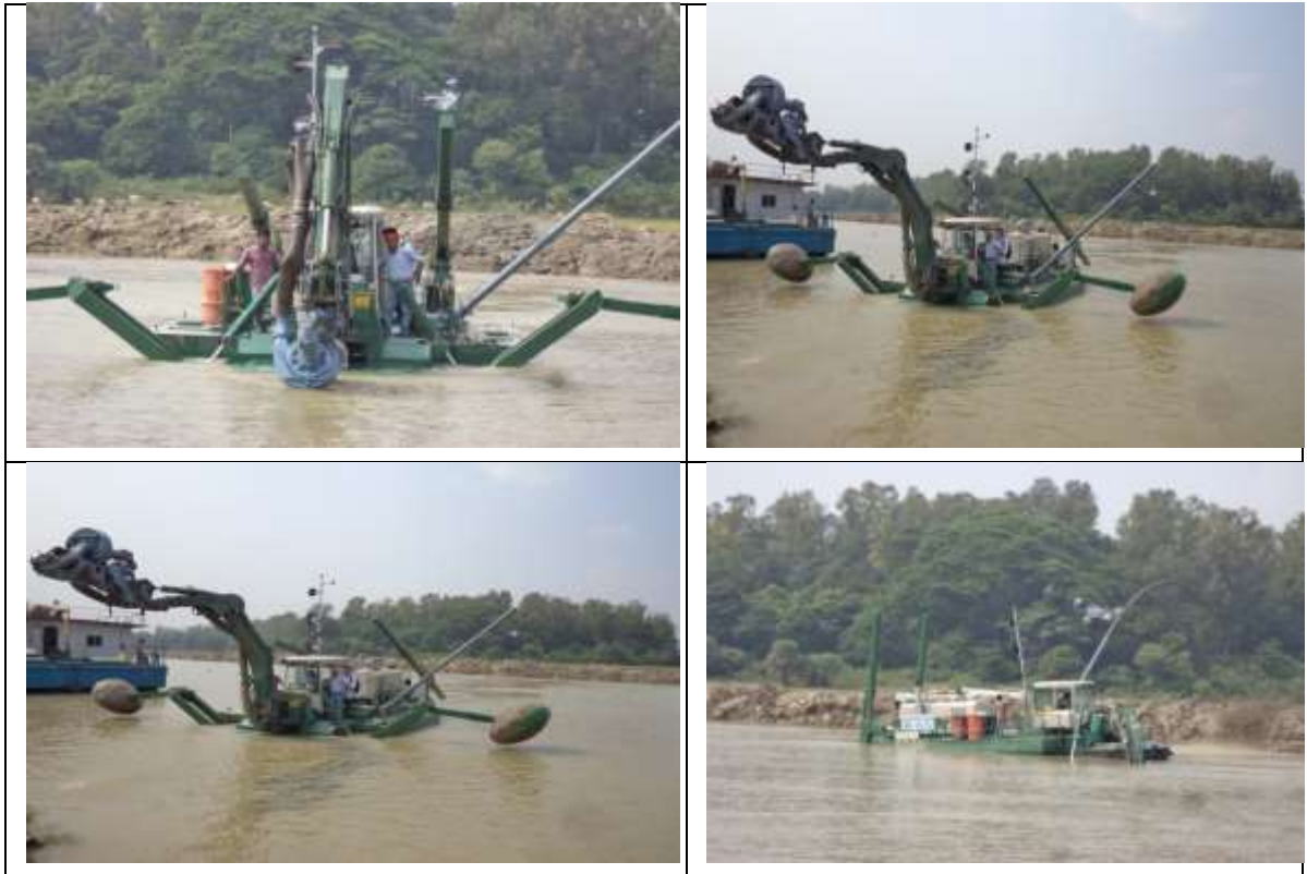
Figure 2.20 : View of Dredging Operations at Farakka
