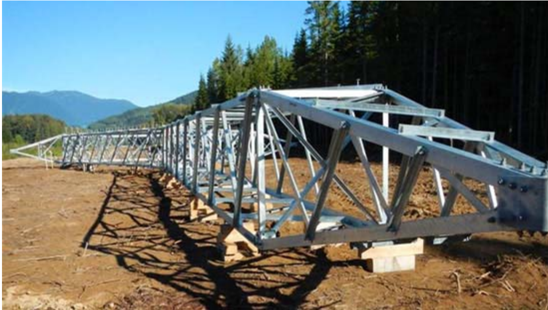
Figure 3.7.2 View of the pole assembled near to foundation
