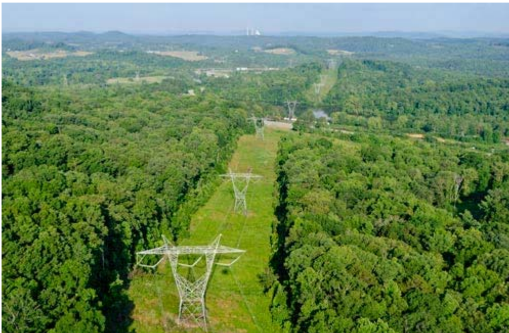
Figure 3.7.3 Example of a cleared corridor in forested terrain
