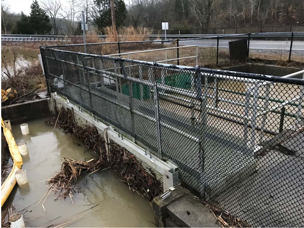
Figure 8.9. K-1007-P1 Holding Pond weir showing debris at the high-water mark and water level of Poplar Creek.
