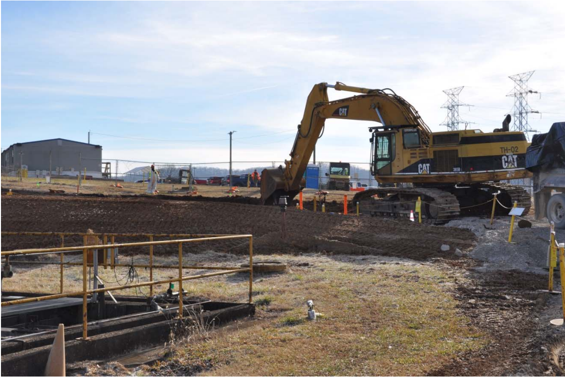
Figure 8.5. Zone 2 EU Z2-12 during remediation.
