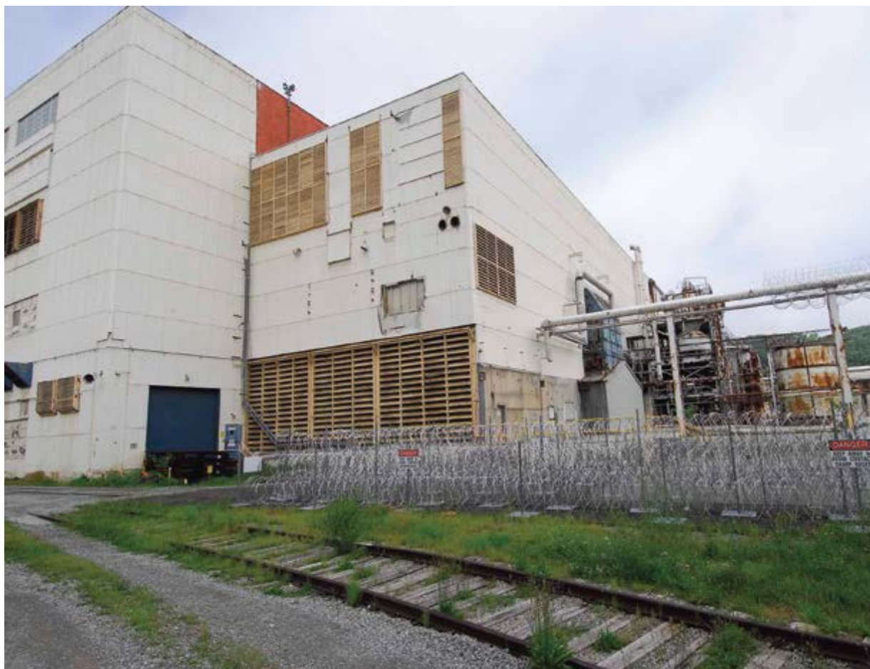
Figure G.1. Colex process pipe located outside on the west side of the Alpha 4 building.
