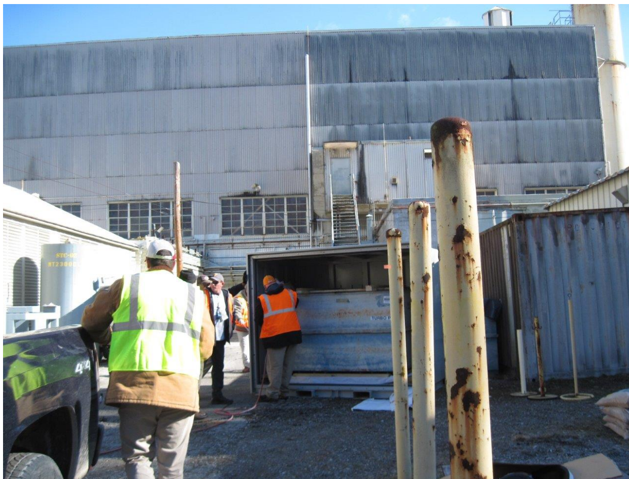
Figure 3.2. MSRE waste being loaded for shipment.
