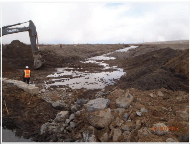
Diversion Channel Construction in Reach T (April 2013)
