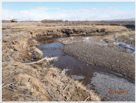
Active Remedial Action in Reach T (May 2013)
