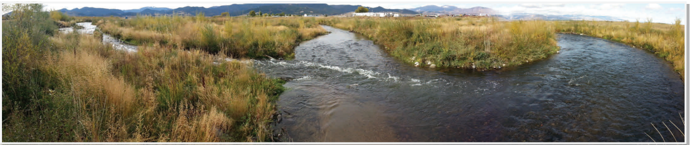
Subarea 4 Recovered Stream Channel - Post 2011 Flooding
