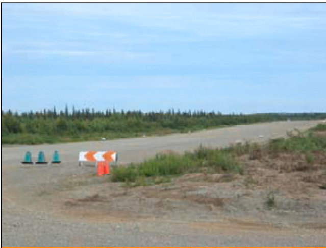
Photo 1 – South end of runway looking north
