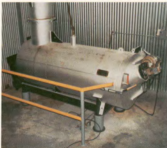
Incinerator used for burning sludge and solid wastes at Camp Lonely. Photograph by Jeep Johnson.
