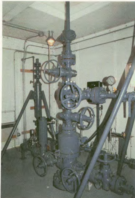
Interior of a wellhouse in the East Barrow gas field, showing a typical wellhead or "Christmas tree" through which the gas is produced. The wellhouses are heated and provide a relatively comfortable environment for the workers. Photograph by Robert Lantz.
