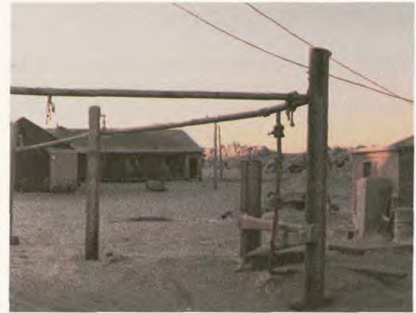
Old gas-distribution system suspended from stanchions. Photograph by Robert Lantz.
