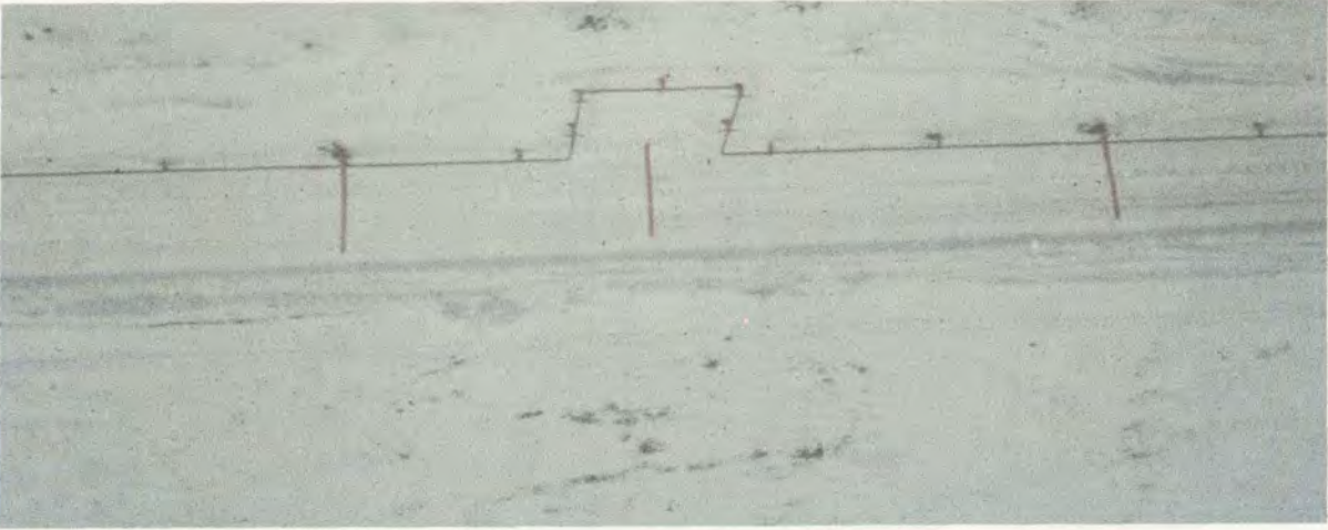
Part of the 6-inch-diameter pipeline from the East Barrow gas field. Expansion loop (center) allows the steel pipe to expand and contract without breaking. The pipe is anchored midway between the expansion loops, which are spaced at regular intervals to avoid any large accumulated movement. The pipeline is supported above ground on wood piling. The taller supports now carry electricity to the East Barrow field. Photograph by Robert Lantz.
