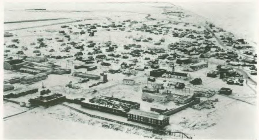
When the Congress approved the sale of gas to the village, a temporary distribution system was built above ground from material left over from the Pet-4 program. Supported on barrel halves or by stanchions, it was prone to leaks and accidental breaks. This photograph of Barrow was taken in 1963 or 1964 during construction of the distribution system. This “temporary” system was replaced in 1982 after some 18 years of service. Photograph by John Schindler.
