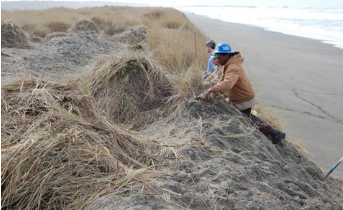
Figure 24. California Conservation Corps working on LEWA/TDSP border to manually remove Ammophila from foredune, in what we now call the “test gap.”
