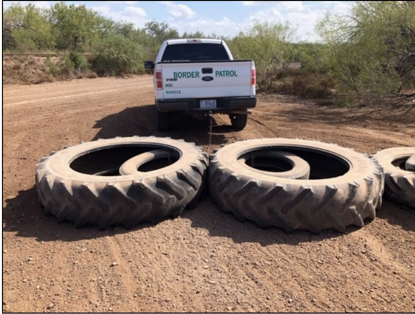
Figure 16. Dragging operations to clear vegetation in ROWs. In some areas, dragging operations extend outside of TxDOT ROWs and into firebreak roads along property fence lines (photograph courtesy CBP, Rio Grande Sector).
