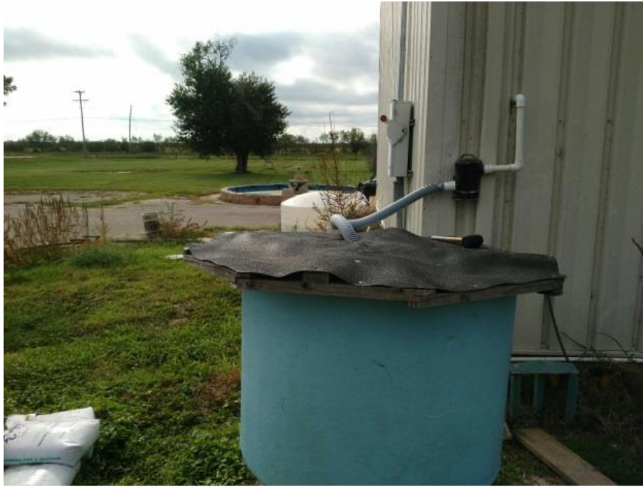
Figure 17. A chlorinated sand filter system at The Uvalde National Fish Hatchery Quarantine Building. Photo credit: USFWS.
