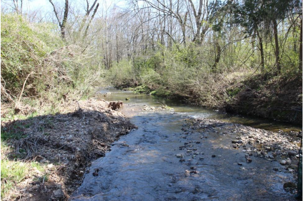
Photo 49. Charles Creek downstream of TN Hwy 287.
