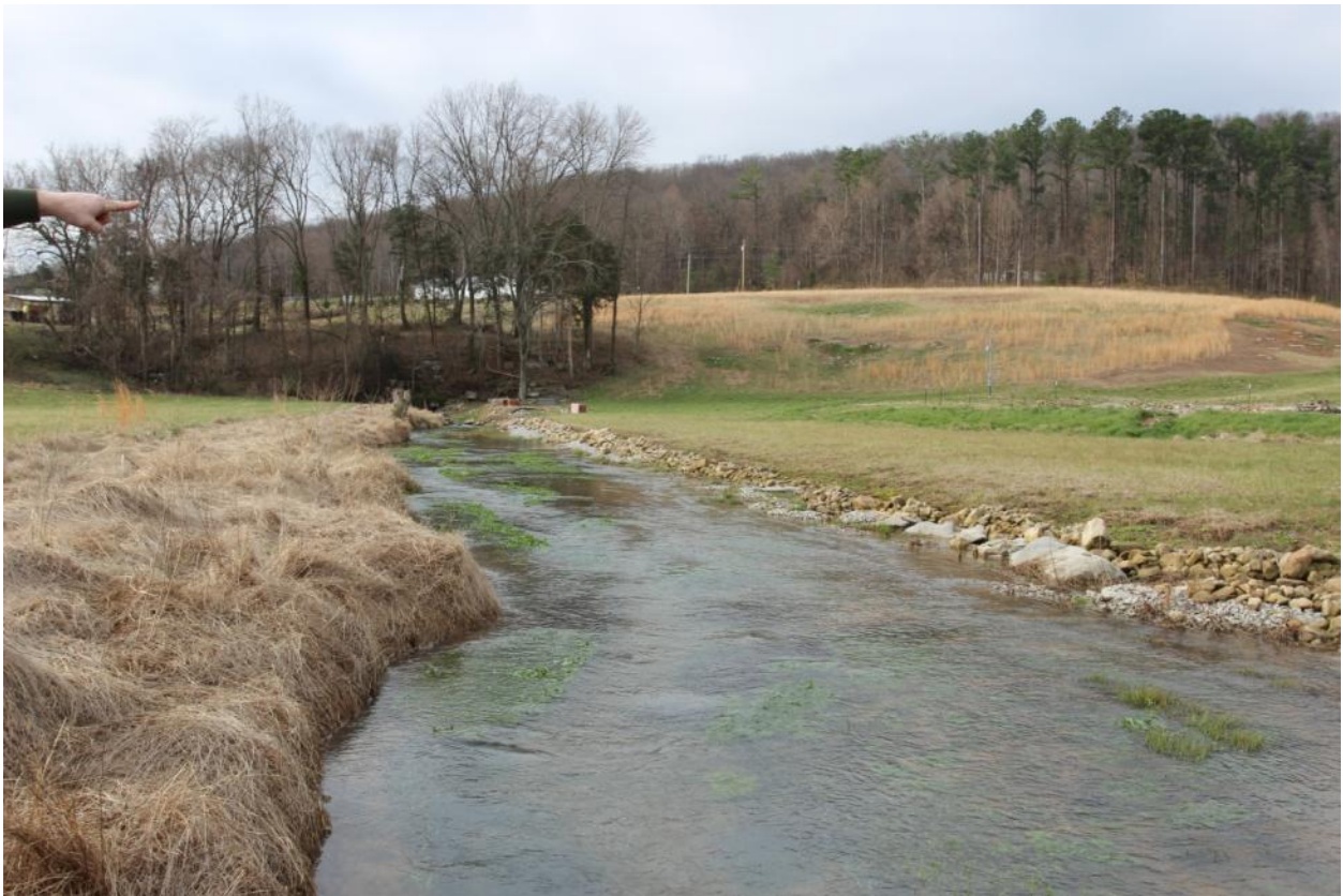
Photo 16. Christian Spring run upstream of Sherwood Road. Note modified run with rip-rap.
