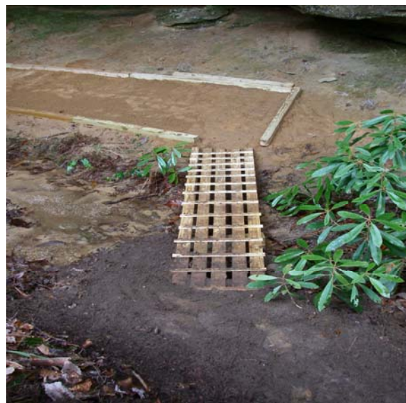
Figure 7: Boardwalk and cribbing along trail.
