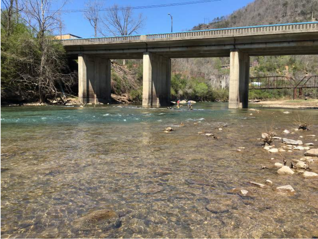
Figure 4: RF2 upstream view
