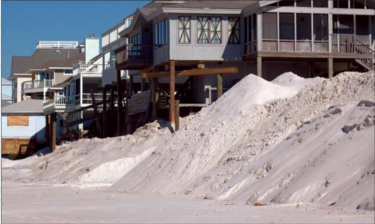
Cape San Blas is one of the quickest eroding beaches in the state. The narrowed beaches and minimal dunes provide inadequate protection to upland property.
