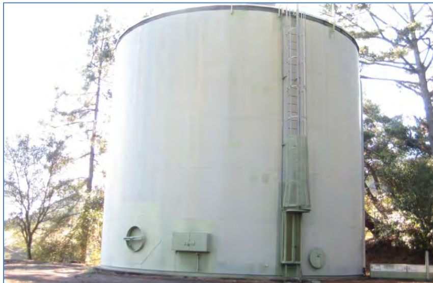
Existing Dos Osos Steel-Welded Reservoir at 8 Los Norrabos in Orinda
