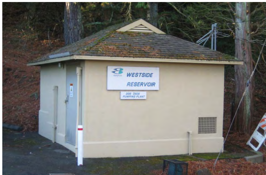
Existing Dos Osos Pumping Plant at 263 El Toyonal in Orinda Figure 2.3
