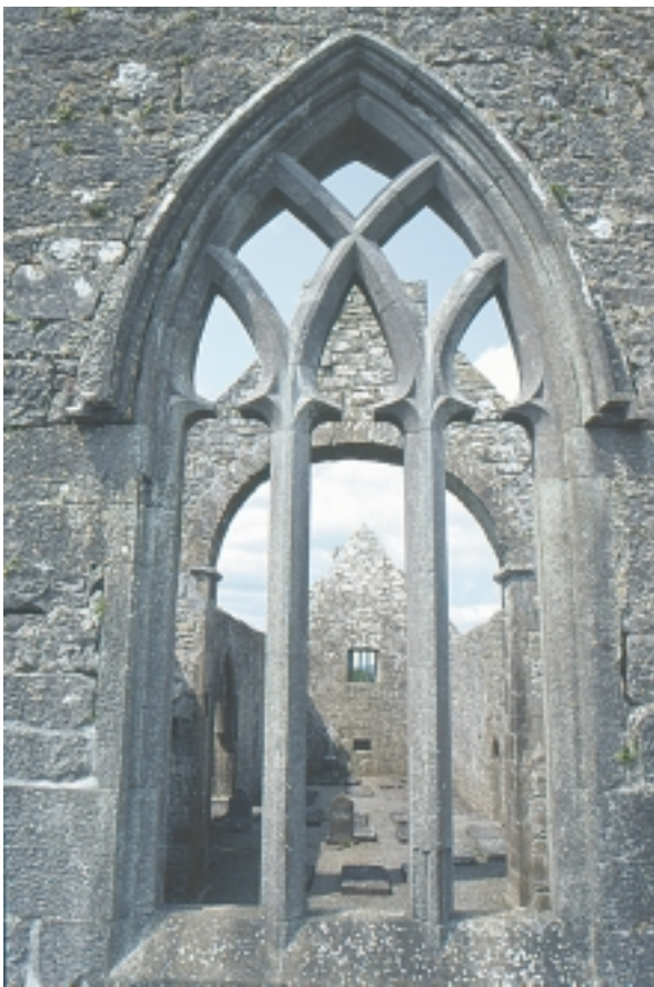
The fifteenth-century traceried east window of Kilmacduagh Cathedral provides a view through to the chancel arch, as well as to the west wall with its late medieval window and simple ancient Irish doorway that was blocked up centuries ago.
