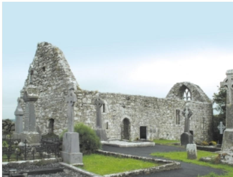
Killursa, the church of St. Furse, was built in two periods, the first comprising the part with the door seen on the left, dating from before 1200, and the second a much expanded structure (with traceried east window) which must have served as a local parish from the fifteenth century.
