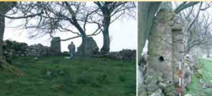
The gateway at the NE corner, with detail of the S wall end showing the aperture for the beam to close the gate as well as the reveal into which the gate sat
