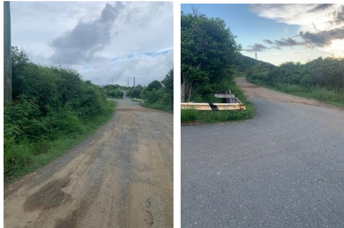
Figure 7.03.1 Photographs of the roadways
