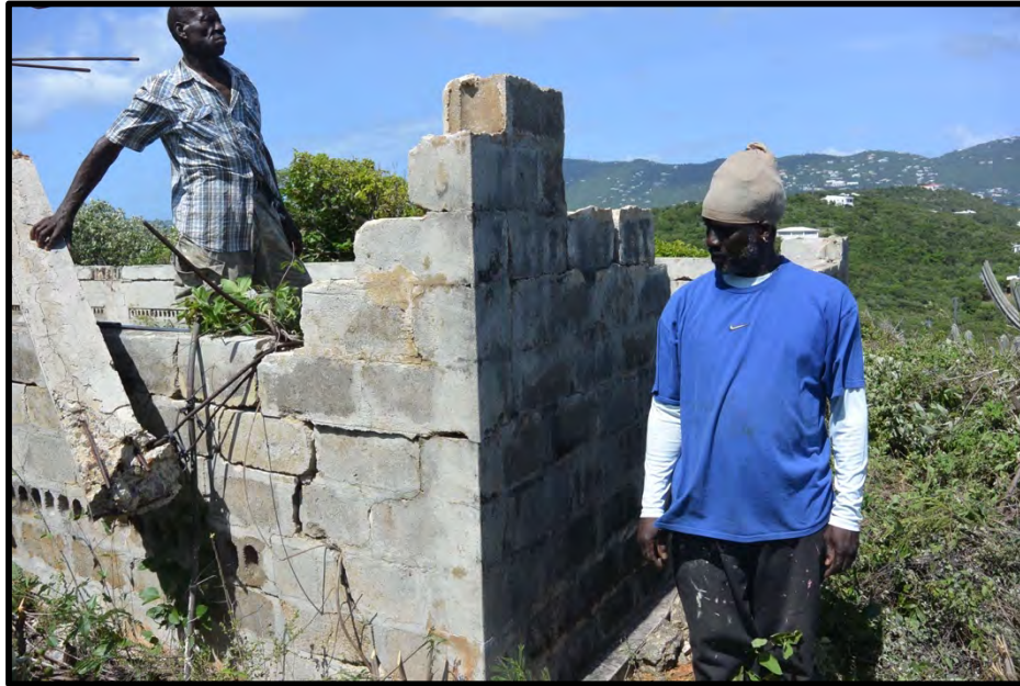
Figure 10: Photograph of the southeastern corner of Building A
