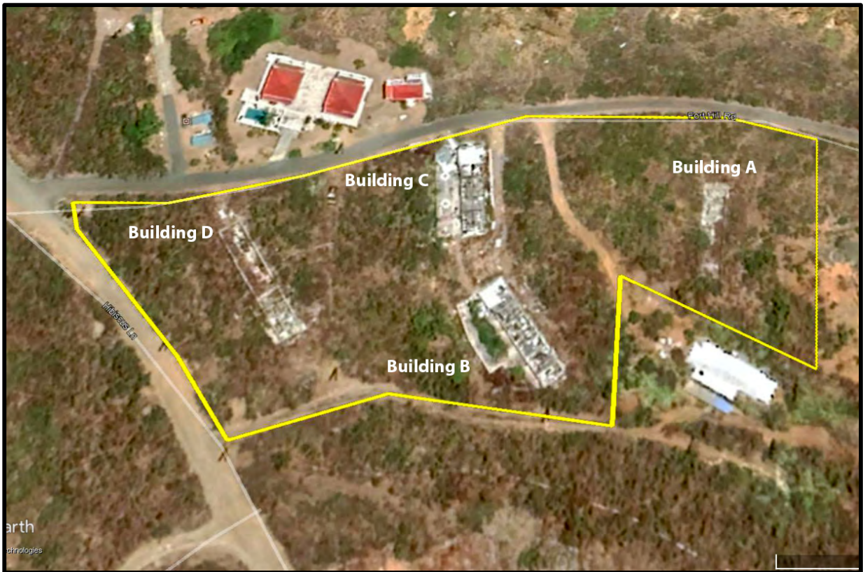
Figure 9: Google Earth image depicting the location of Buildings A – D)
