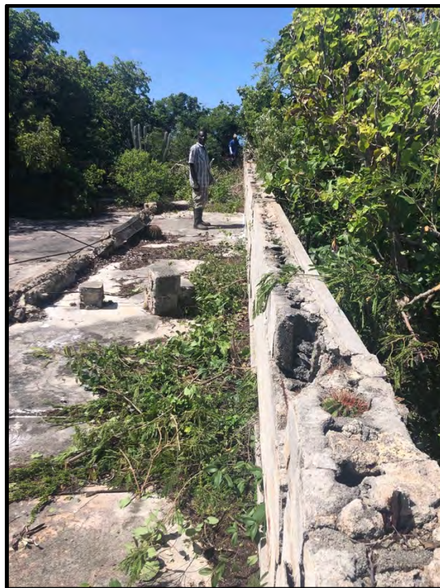
Figure 11: Photograph of the north wall axis, view to the west
