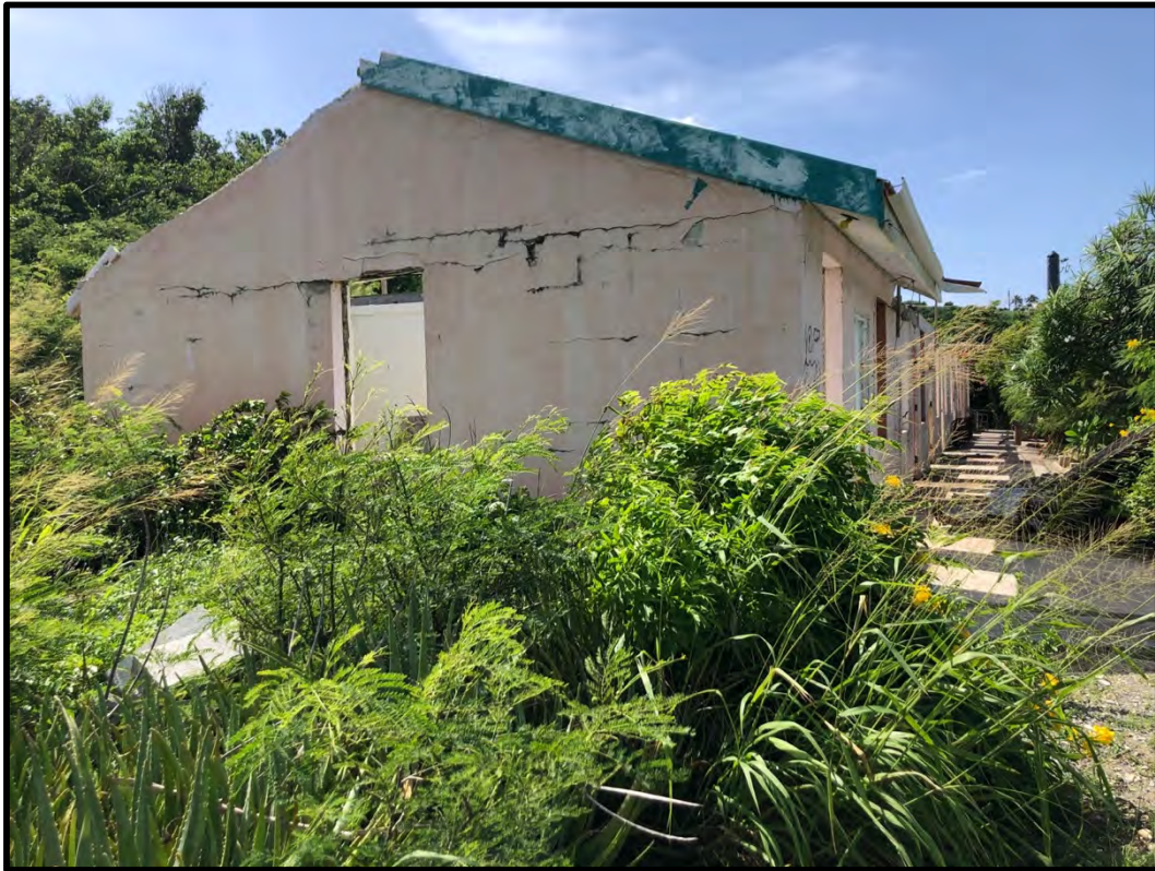
Figure 14: East elevation of Building B
