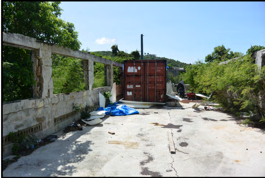
Figure 19: Building D interior, view to west
