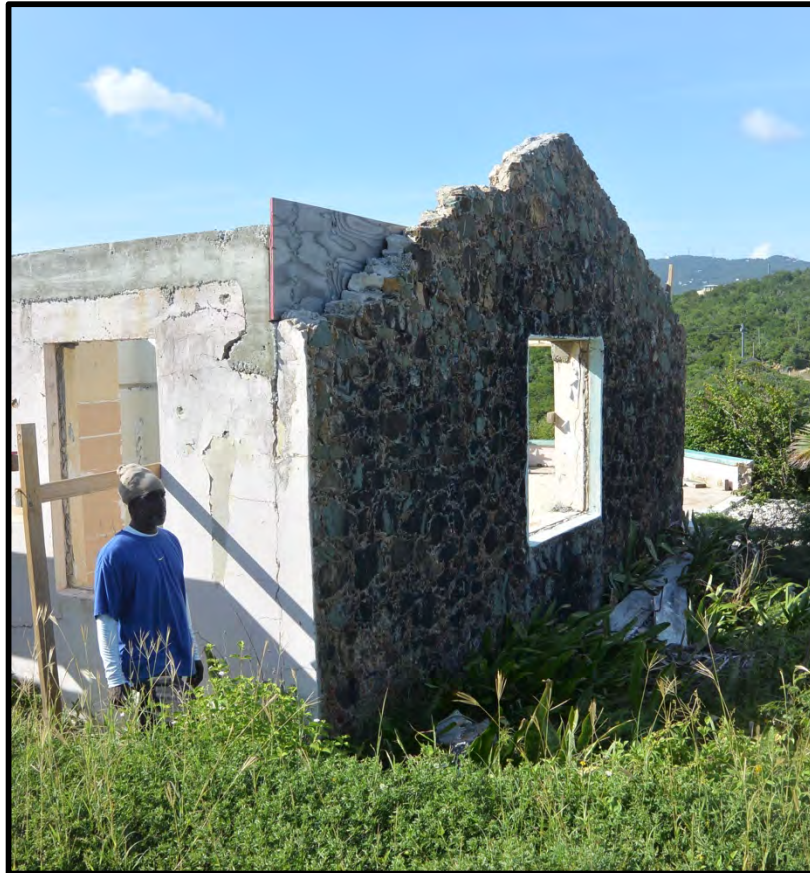
Figure 18: Rock faced east elevation of Building C
