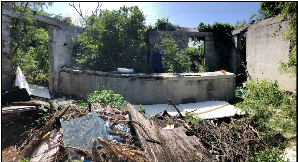
Figure 20: Photograph of the west end of Building D
