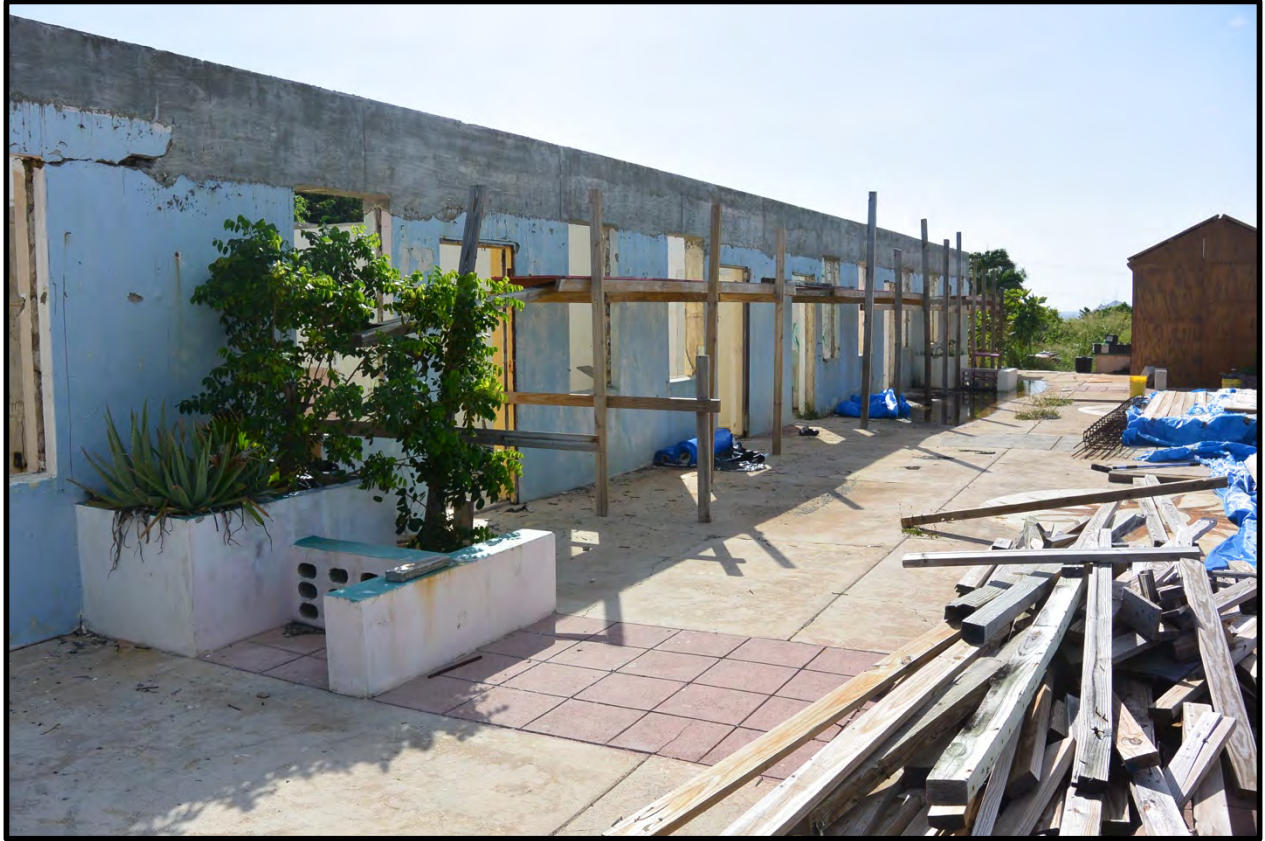
Figure 18: Partial view of the north elevation of Building C
