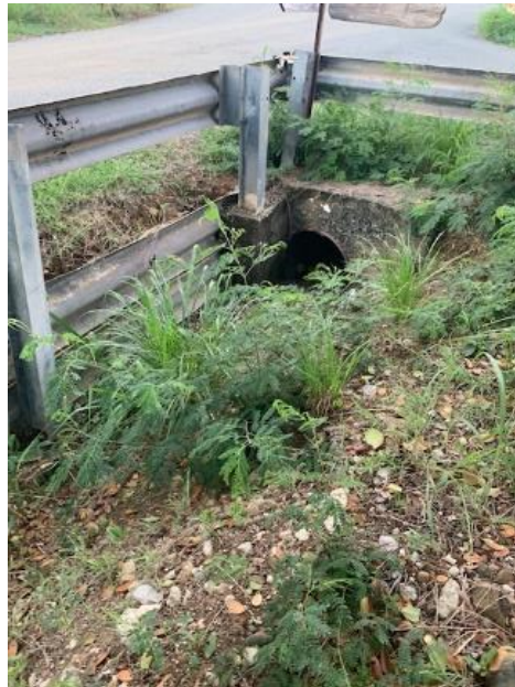
Figure 6.03.2 Existing culvert on proposed project site
