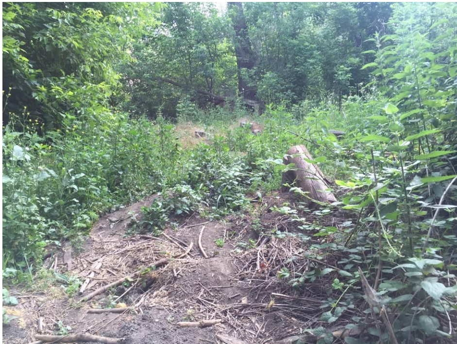
Figure 11. Cut down tree and stockpile of wood.
