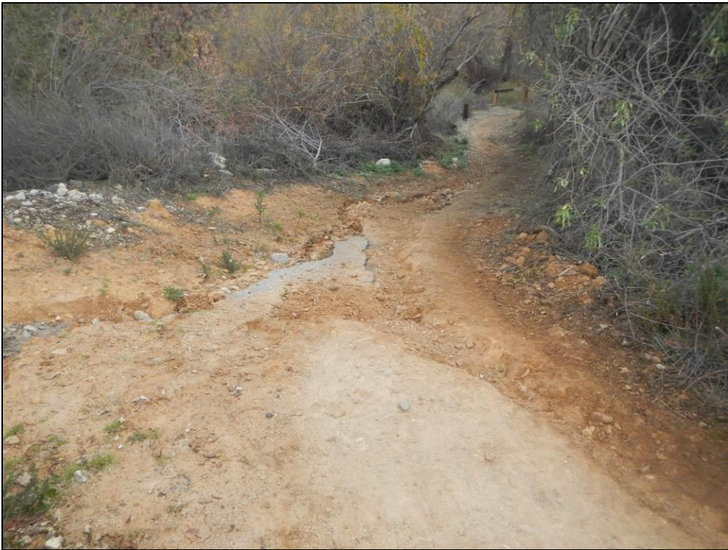
Figure 14. Eroded trail leading from cottonwood upland area to Haines Canyon Creek on January 18, 2016.
