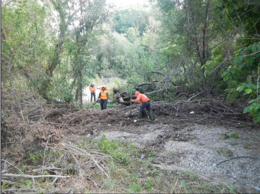
Figure 9. Crew using chainsaw and hand tools to clear fallen tree and debris obstruction from trail.
