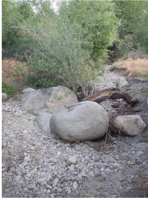
Figure 8. Heavy erosion and large boulders blocking trail.
