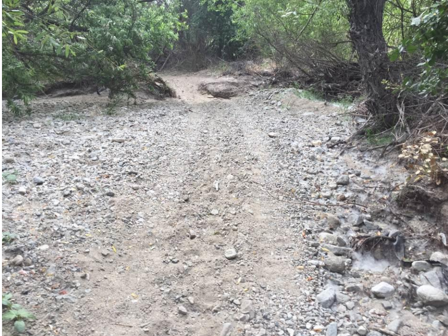
Figure 10. Evidence of ATV use on trail.
