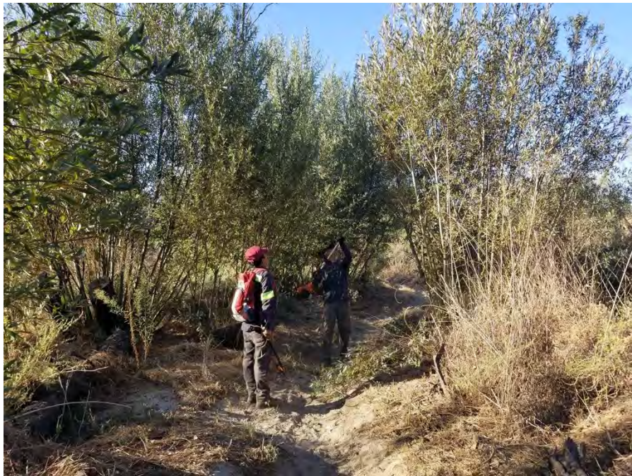
Photo 8. As the crew approached the western trail alignment, they trimmed overhanging willows that impeded the trail making a less navigable route for equestrians, on October 30.
