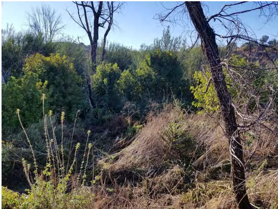
Photo 14. After the patches of white sweetclover and shortpod mustard were cut using weed whippers and tree of heavens and castor beans were removed using shovels to remove root structures to reduce the potential for regrowth, on October 16.
