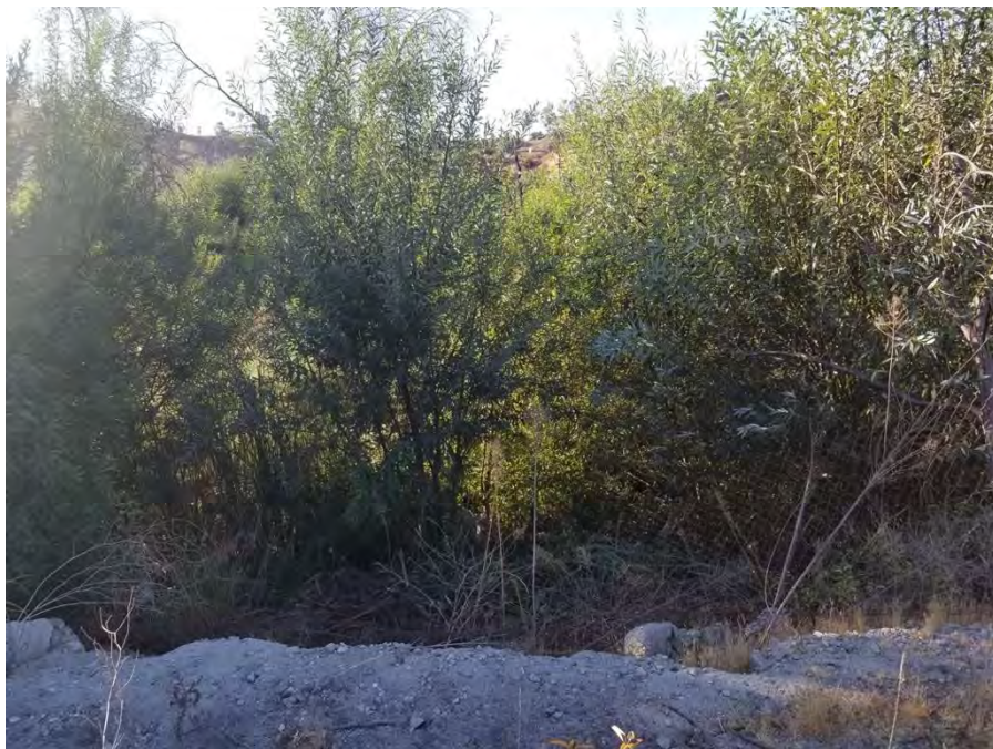
Photo 18. After the careful removal of the castor bean patch using shovels, to minimize soil deposition into the creek, on October 19.
