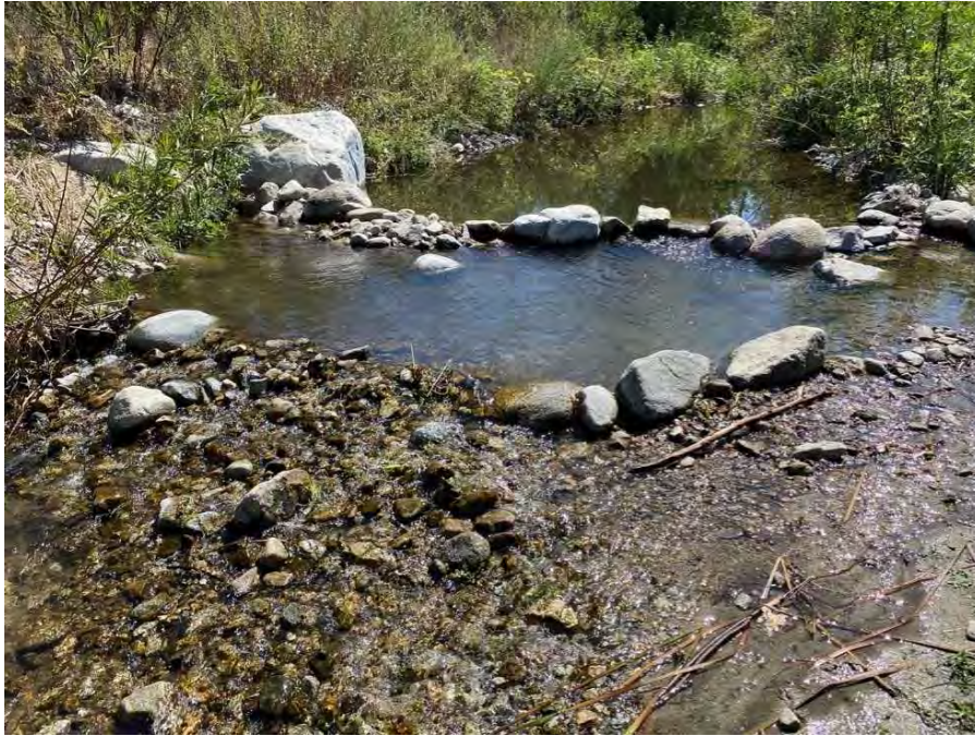
Photo 1: Illegal dam composed of large rocks and boulders observed on August 30, 2020, during a public outreach effort. The dam was located along Haines Canyon Creek northwest of the south Wheatland Avenue entrance.
