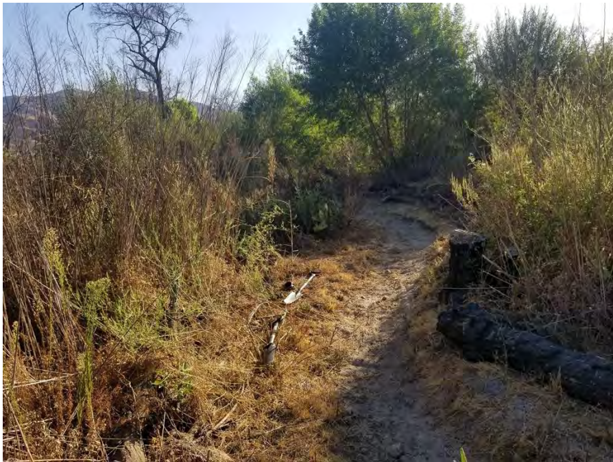
Photo 4. The crew used weed-whippers to clear the trail and trim back vegetation at a margin of 4 feet, on September 28.
