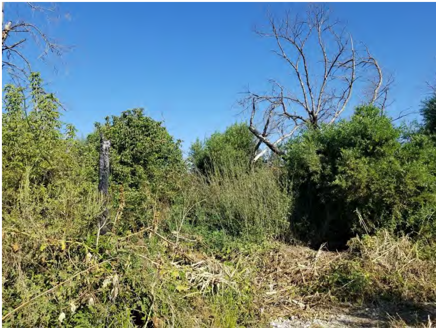
Photo 12. After the removal of castor bean using machetes and shovels to remove root structures to reduce the potential for regrowth, on September 30.
