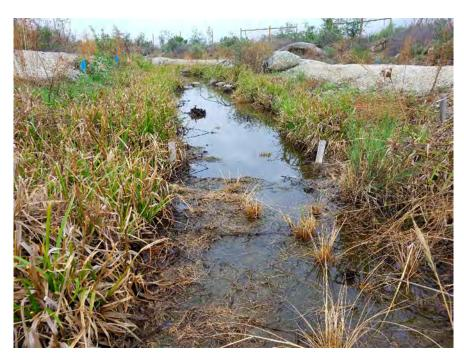
**March 2018.** Ephemeral flows occur in the designed spiraling drainages that convey off-site/on-site flows to an outlet tower in the center of the Lower SPS.
