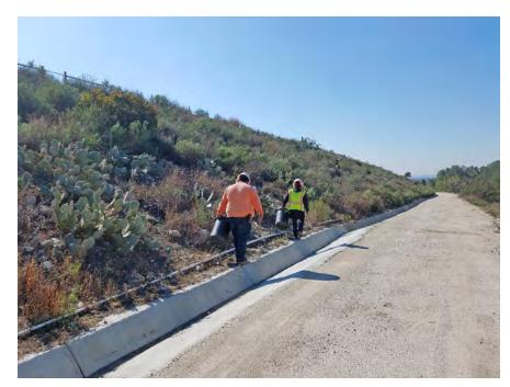
**February 2018.** Maintenance tasks include the inspection of concrete drainage structures, and the removal of sediment and debris to maintain the integrity of storm flows through the Lower Sediment Placement Site (SPS).
