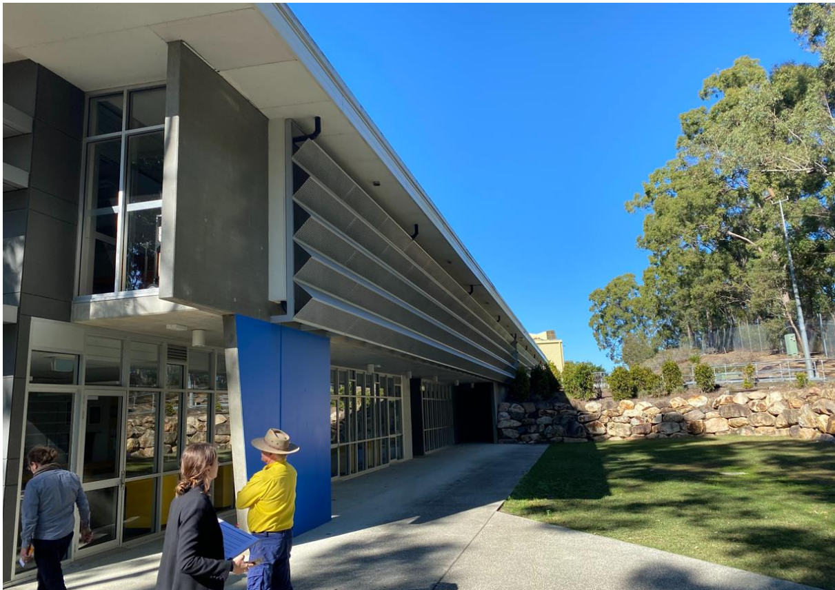
Figure 5-12 Interface with Western Boundary of the College (Army Barracks) Source: Urbicus site photos
