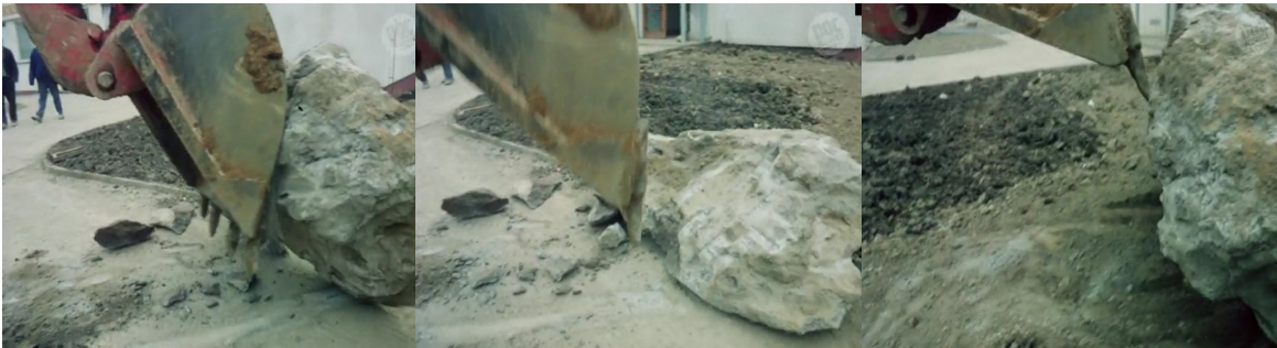
Figure 30: Excavator pushing a rock ( Panelstory )
