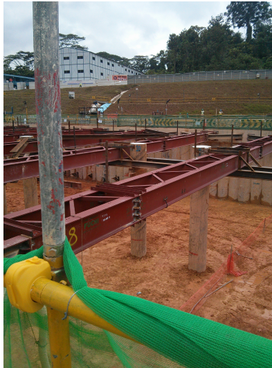
Figure 6: Excavation pit being prepared for the insertion of Level 2 struts.
