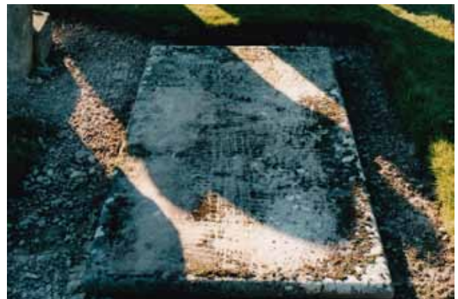
Figure 98: The moss from this gravestone has been removed using a rake. © Susan Buckham
