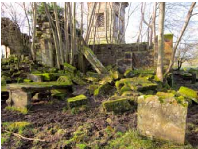
Figure 96: View showing the poor condition of the landscape at St Michael's Churchyard, Cambusnethan, North Lanarkshire. The graveyard, along with three mausolea, is Category B listed. The graveyard contains several late-medieval grave-slabs and an early medieval cross-shaft was discovered here in 1898. © Susan Buckham
