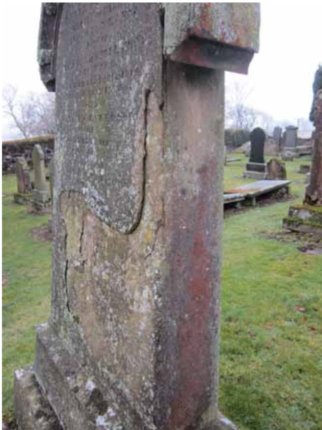
Figure 49: Delamination on sandstone headstone, Glassford Churchyard, South Lanarkshire. This burial site was surveyed to assess its cultural and natural values as part of the Clyde and Avon Valley Landscape Partnership’s graveyard conservation strategy. © Susan Buckham
