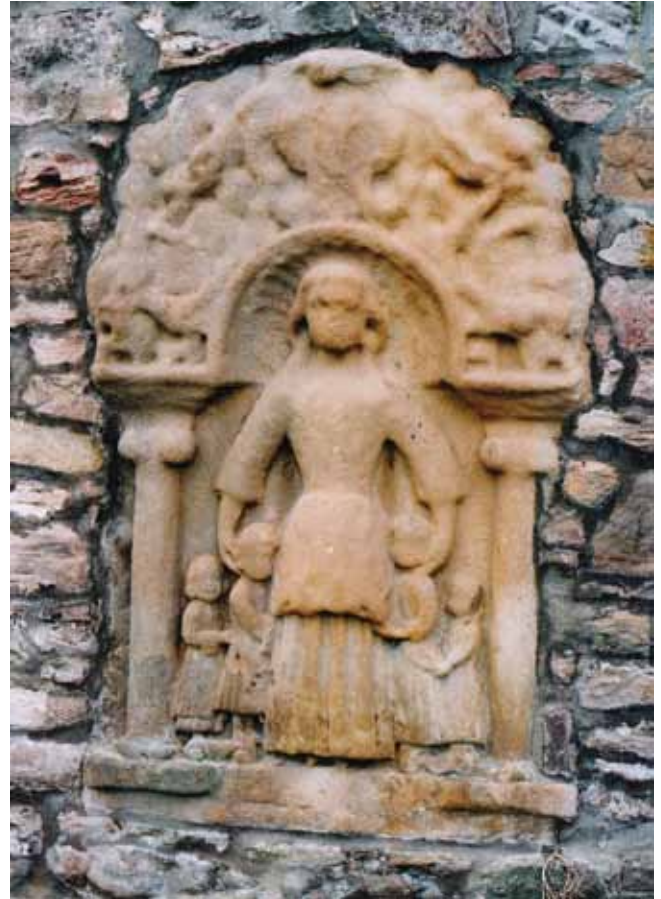
Figure 90: A sandstone headstone suffering from severe stone decay. This stone was moved and reset into the boundary wall of Preston West Churchyard, Prestonpans, East Lothian. © Susan Buckham
