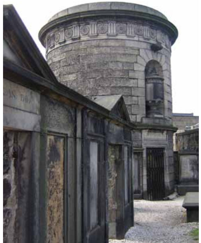
Figure 53: Circular mausoleum of David Hume and distinctive row of walled burial enclosures, Calton Old Burial Ground, Edinburgh. © Susan Buckham
