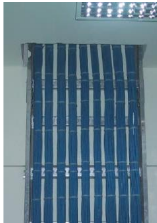
Figura 3.5: Cableado Vertical
