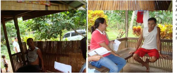
*Left* –crushed bamboo used as walls *Right* – 35-yr oldbamboo floor shows no signs of deterioration *Below* – Bamboo seats are common house fixtures
