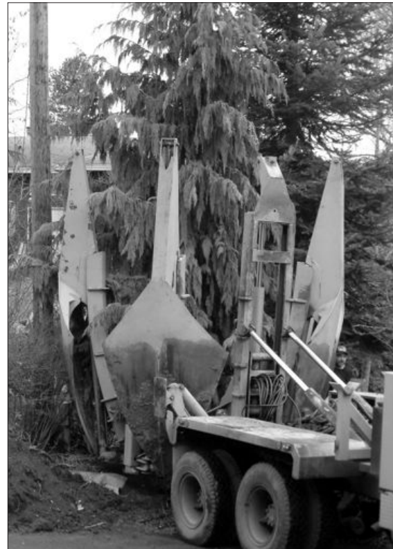
Careful alignment is required to center the tree and preserve as many roots as possible.
